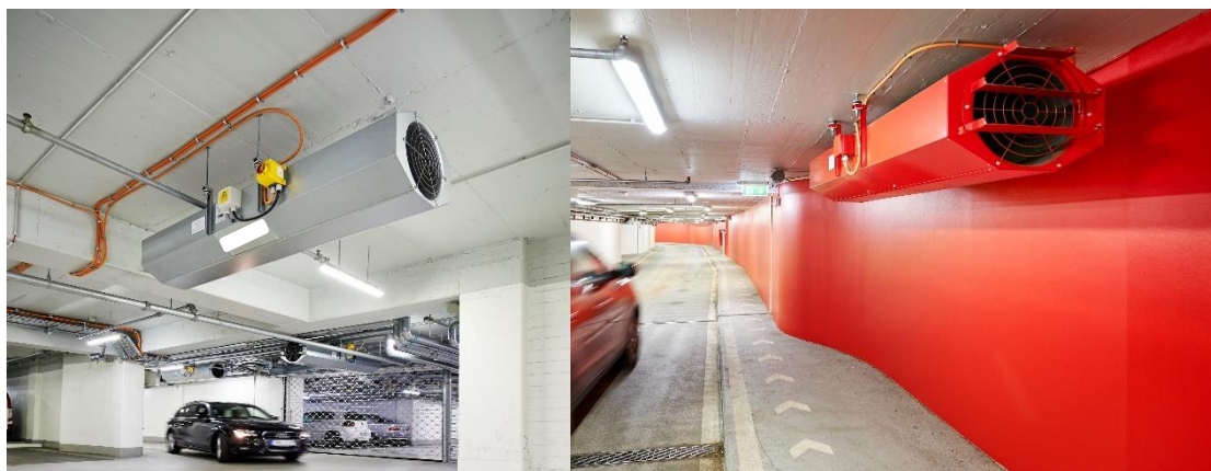
Figure 6 - example of the use of Jet Fans for enclosed car park ventilation
