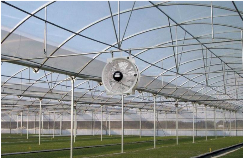
Figure 10 - example of the use of a large circulating fan with a stator in a horticultural application
