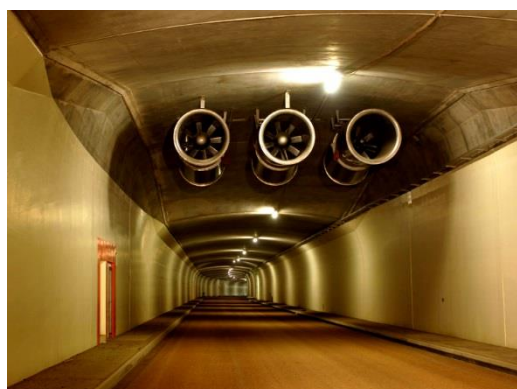
Figure 5 - example of the use of Jet Fans for tunnel ventilation
